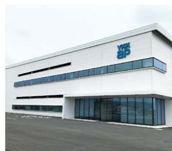
Saitama Factory new building
